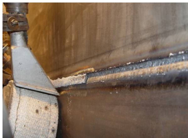
Fig 1- 2: SAW process on horizontal joint
