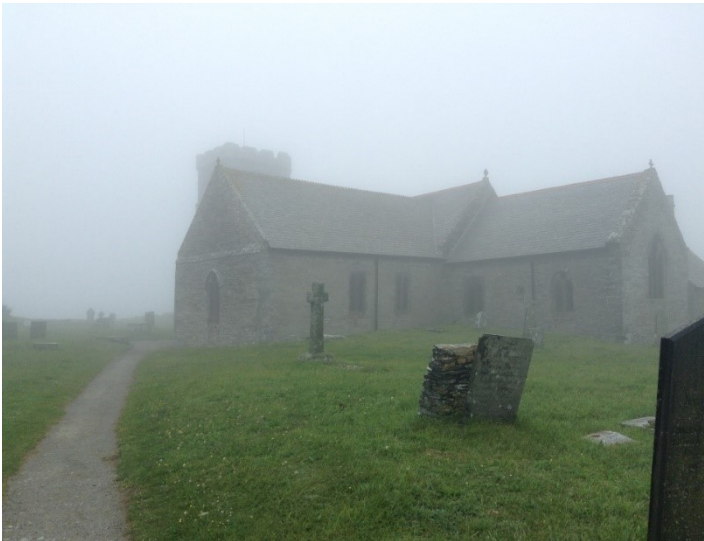
Figure 3.7. Exterior of St. Materiana's Church, Tintagel.
