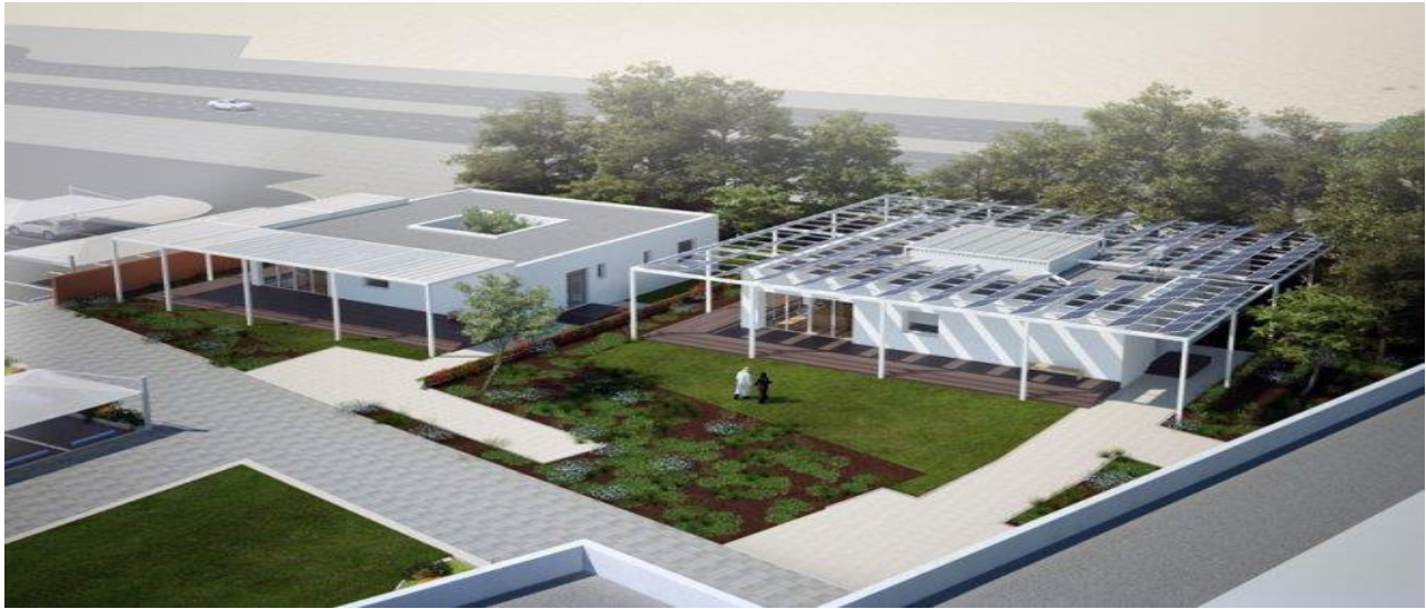
Fig. 1.2. Concrete passive house for two families in Qatar
