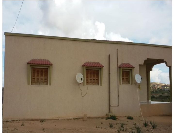
Fig.2.2. The South Façade
