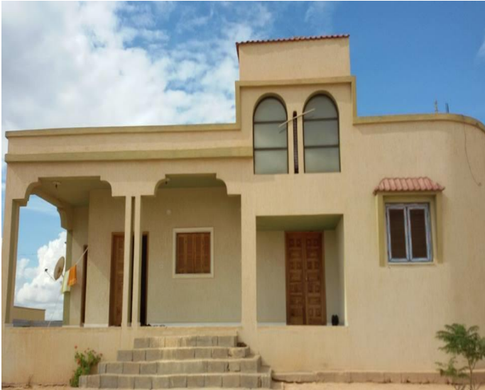
Fig.2.1 The Front Façade
