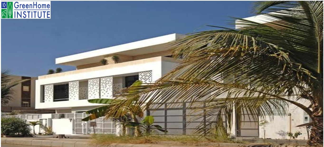
Fig. 1.4. Concrete passive house built in Saudi Arabia
