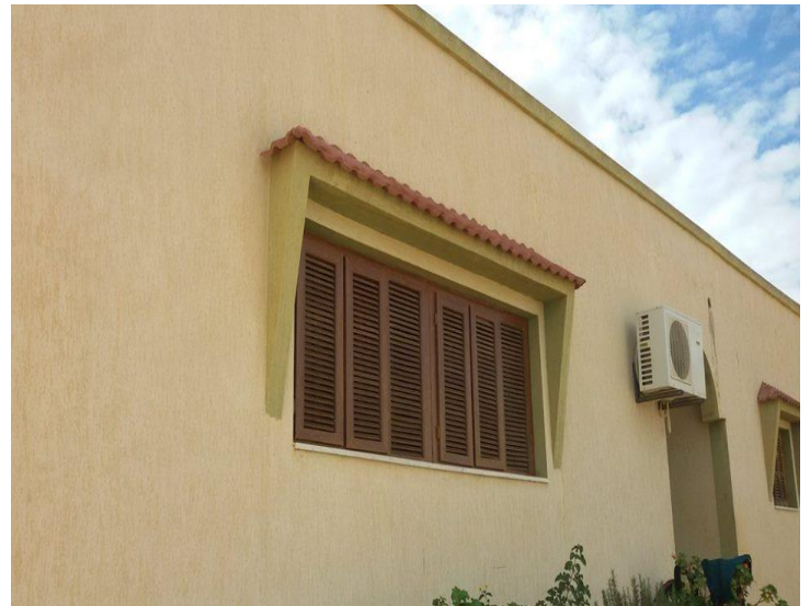
Fig. 2.4. The North Façade
