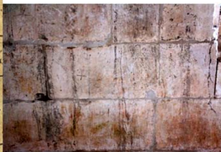
Fig. 2. Constructing traces left by medieval masons on the cloister wall of Batalha Monastery (Batalha, Portugal) (Authors' photo)
