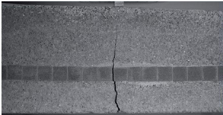
Figure 9 - Concrete sample, one big crack visible [11].
