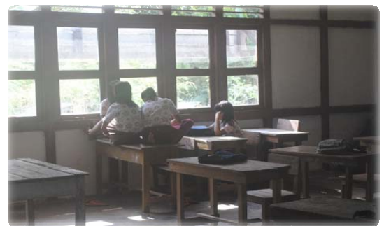
Fig. 3 The condition of classrooms
