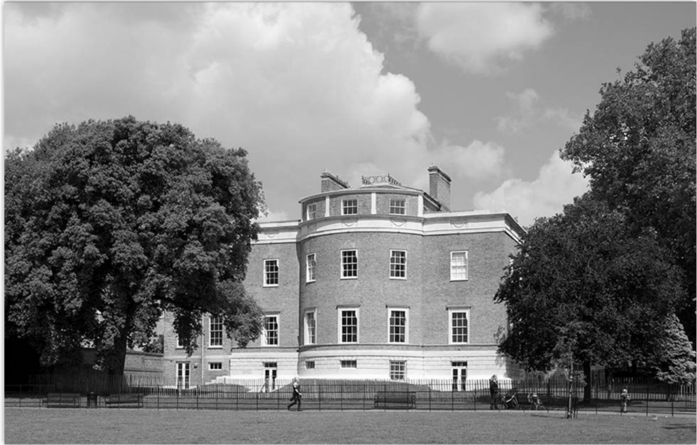
Photography 5. Manor House Library
