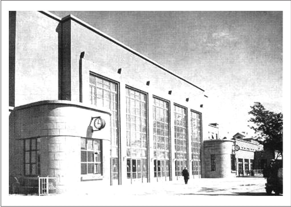
Figure 12. Entrance from the platforms.
