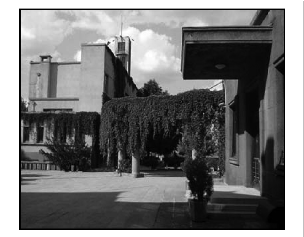
Figure 10. Joint between the station building and the casino building. Source: Photograph taken by Segah Sak.
