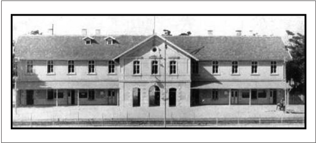
Figure 7. The facade of the old train station seen from the railway.
