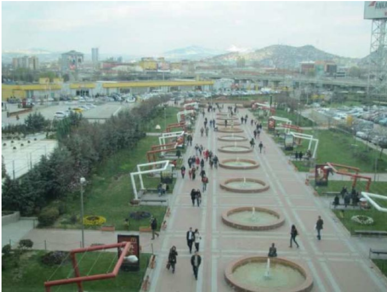
Figure 2. View of the ANKA mall Park and Akköprü metro station from ANKA mall.
