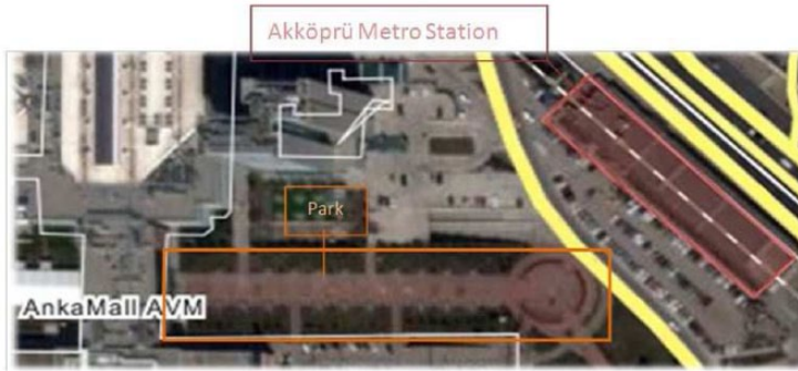
Figure 1. Site view of Akköprü metro station, Turkey.
