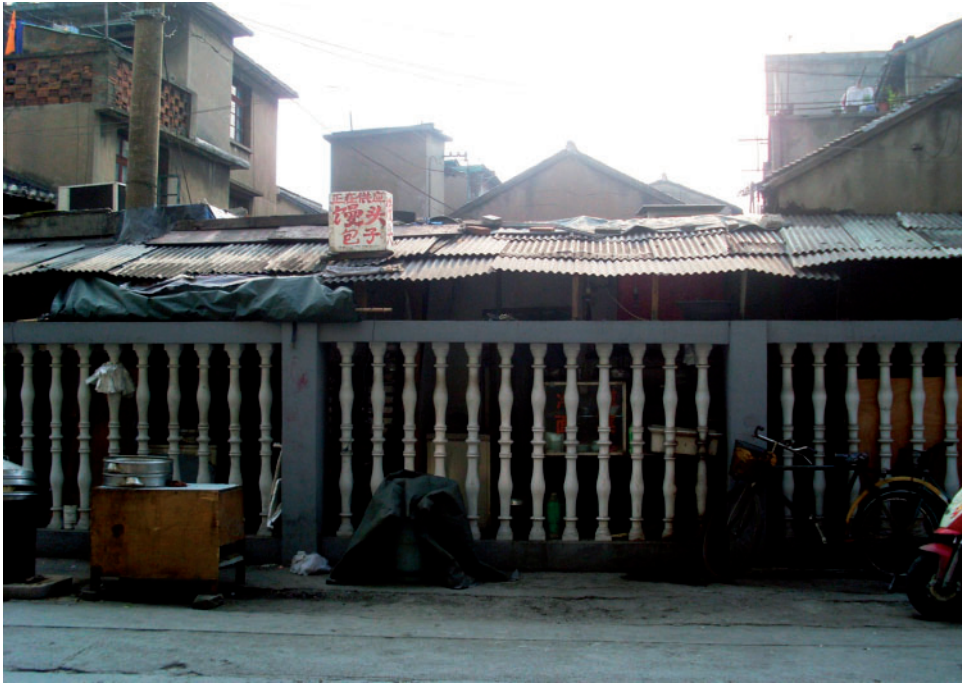
Figure 1. Work-live Arrangements behind the Concrete Fence. Shanghai, 2008. Photograph: Deljana Iossifova.
