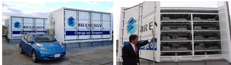
Figure 3.3: Images of the demonstrator 4R-energy wind farm energy storage project in Osaka, Japan.
