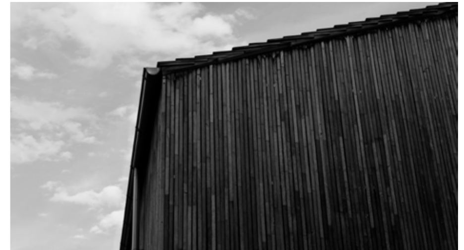
Figure 2. Peter Zumthor, Atelier, Haldenstein, 1986. Detail of the outer skin.
