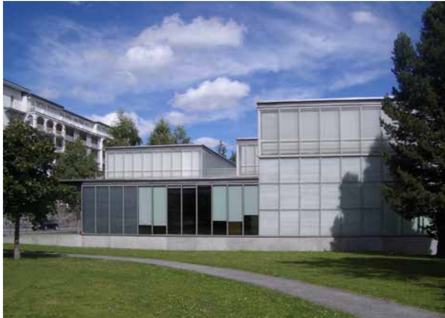
_ Figure 7. Gigon & Guyer, Kirchner Museum, Davos, 1989- 1992. On the outside the envelope remains indecipherable: the translucent surface of the glass creates a sense of indefinite depth; however the glass sheets provide visibility of the underlying whitish fibre-glass insulation, thus making the stratification evident.
