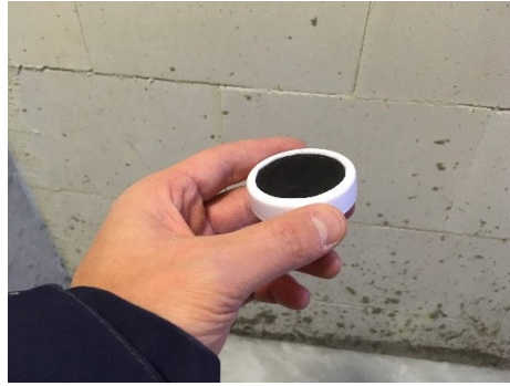
Figure 61 The Gore-Tex membrane was replaced
