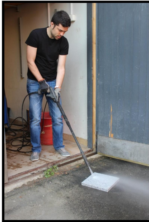
Figure 6-7. Cleaning the granite stone.
