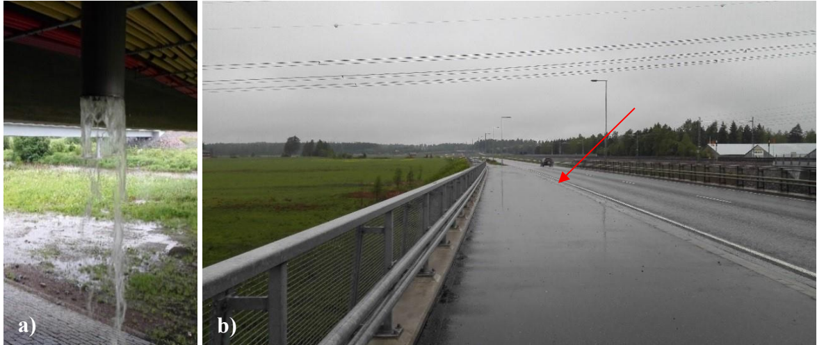
Figure 11. The downspout (a) of a bridge (b) used for untreated stormwater sampling. Location of the inlet of the downspout is denoted with red arrow. The actual test site is ca. 250 m away.
