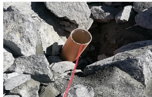
FIGURE 22: CARTBOARD PROTECTION OF DRILLHOLES
