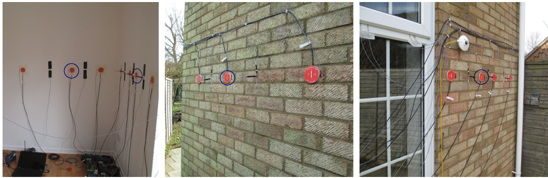
Figure 4. Internal (left) view of the north- and east-facing walls (with the north-facing one on the left side of the corner), external north-facing wall (middle), and external east-facing wall (right) for the cavity wall (CWall) case study. The pair of sensors analysed are circled in blue.
