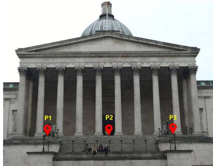
Figure 6—Intermediate environment data collection sites on the portico of UCL's Wilkins building
