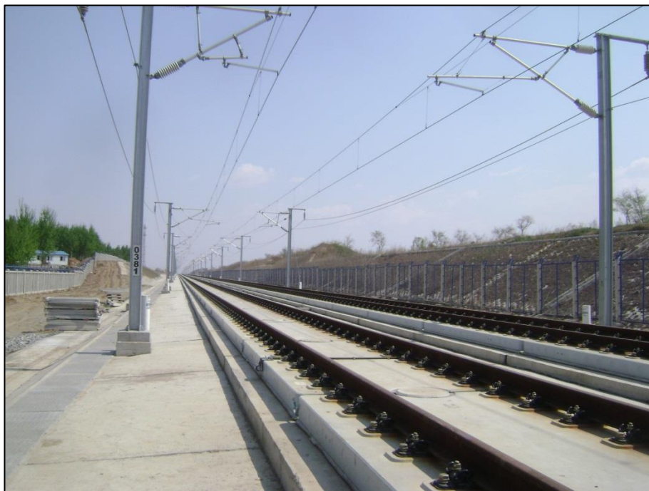
Fig 2.4 Shinkansen slab track on Ha-Da PDL of Northeast China
