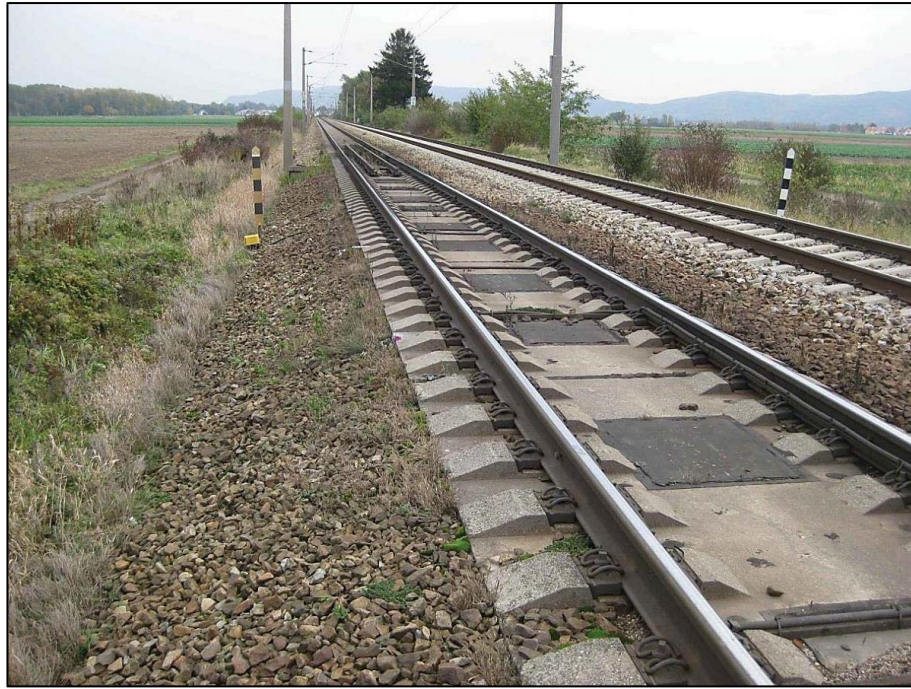
Fig 2.8 ÖBB–PORR in Langenleobarn, Austria (Pichler and Fenske, 2013)
