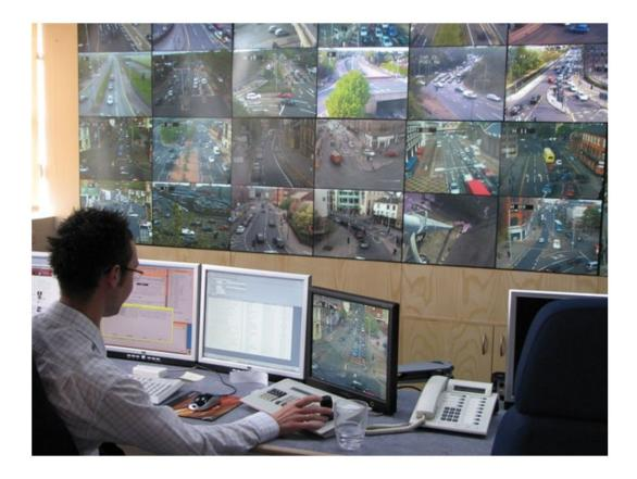
Figure 1.1: The urban traffic control system monitors more than 450 of the intersections in Nottingham (Source: World Highways, 2010)
