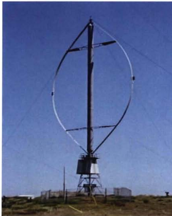
Figure 8: A traditional Darrieus troposkein VAWT. (Courtesy of Wikipedia)
