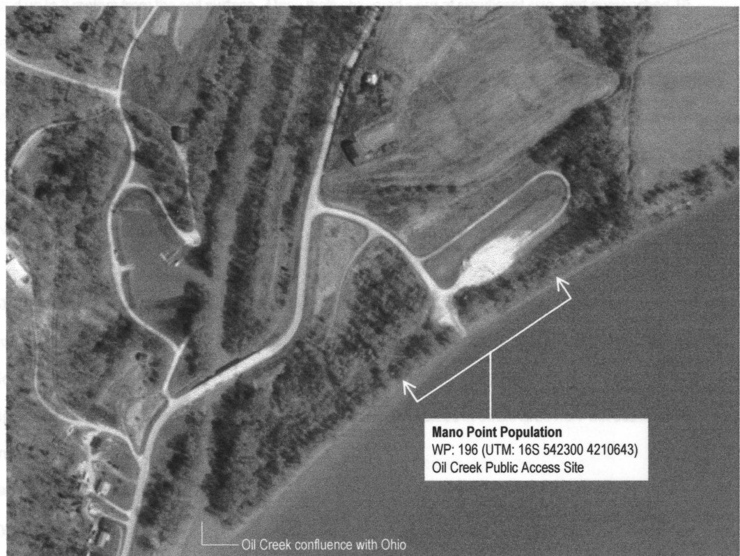
Figure 24. Digital orthoquadrangle of the Mano Point Ohio River Access Site near Derby, Indiana
