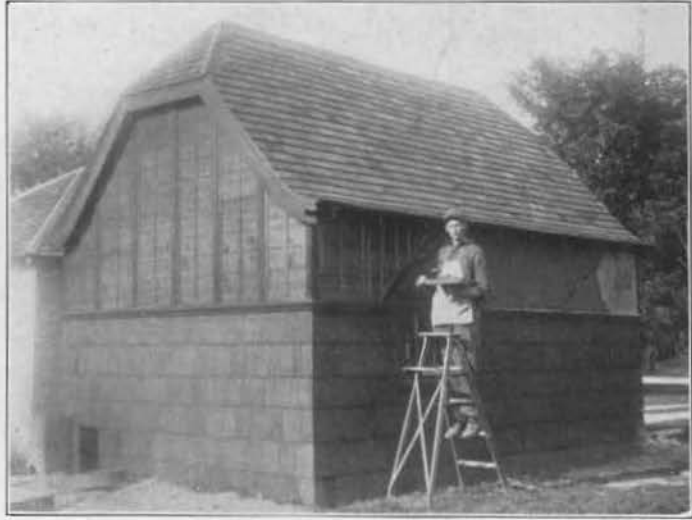
Student, Plastering Upper Part of Garage Which He Built. At Left May Be Seen the Finished Building
