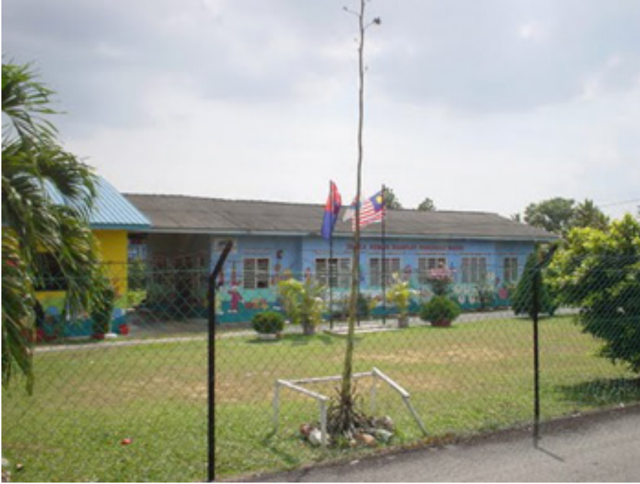
Public preschool building in a rural area
