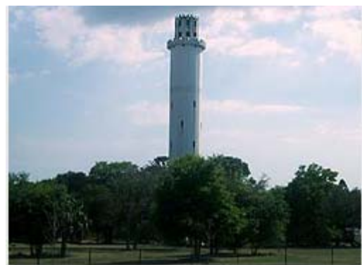
Figure 3. Sulphur Springs Water Tower
