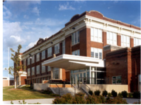
Fig 45 restored elementary school
