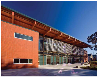
Rosa Parks School at New Columbia Community Campus Location: Portland, Ore. Architect: Dull Olson
