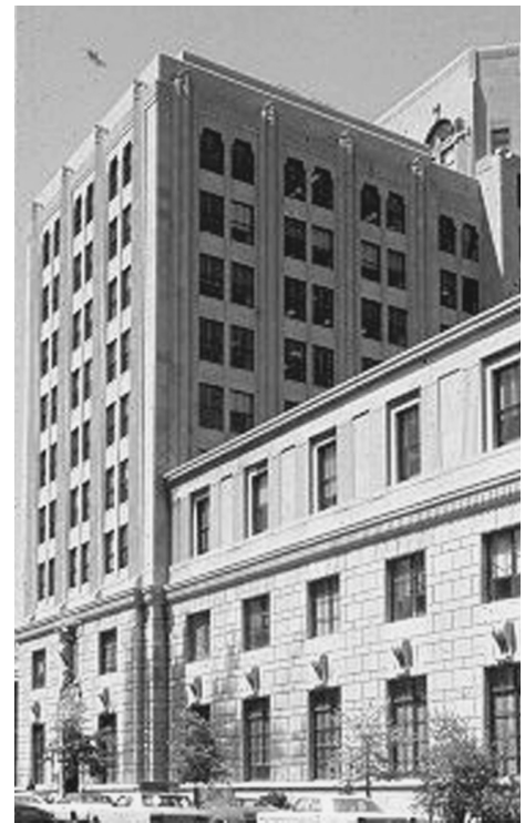
Fig. 21: Civic Landmark: School Administration Building, 1931
