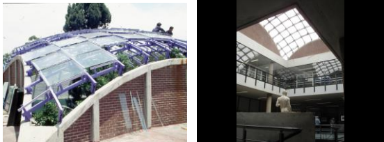
b) Hall of the Faculty of Architecture at University of Mexico, Mexico City, Juan Gerardo Oliva, 1992
