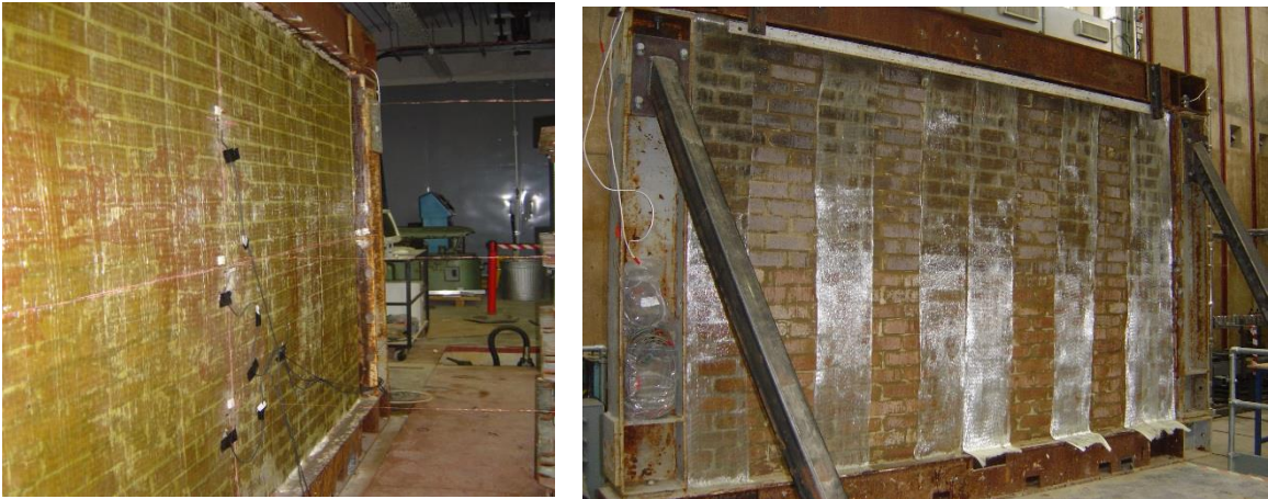
Figure 2 FRP reinforced panel with 100% RR (left) and panel with 60% RR (right).
