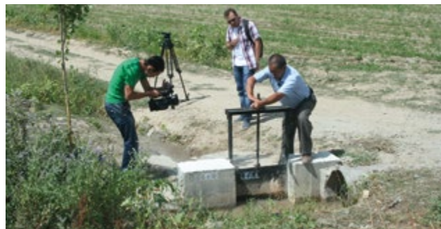
Farmers – beneficiaries of the project on rational use of water resources in the south of Kyrgyzstan – demonstrate work of sluice gates in the field. (OSCE/Svetlana Levina)
