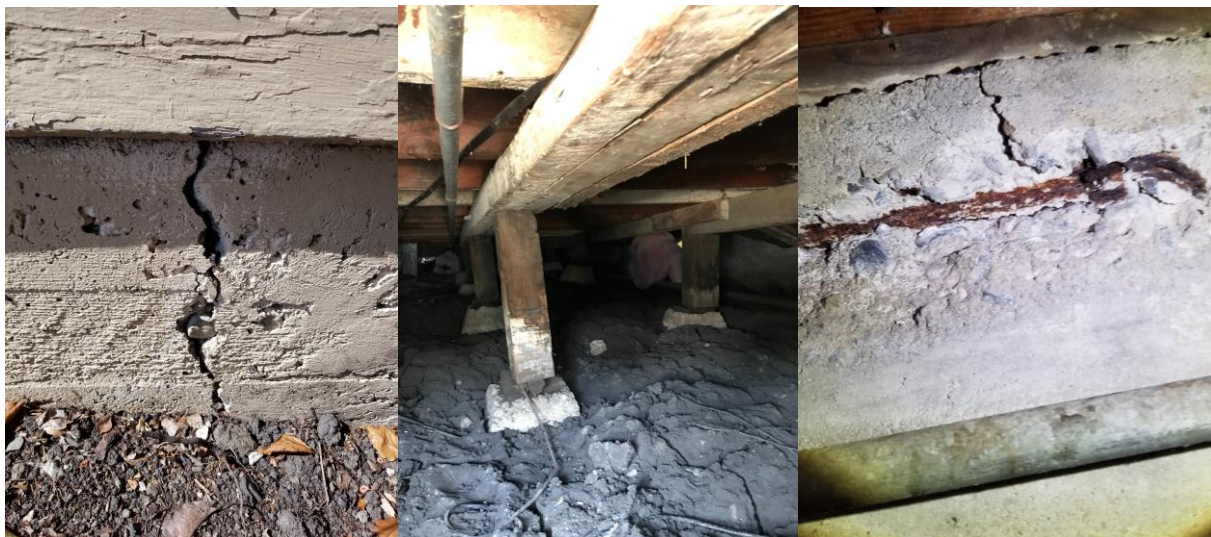
Figure 1: Condition of Existing Foundations
