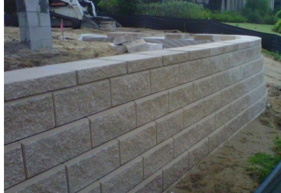
Figure 6: Typical Allan Block Retaining Wall
