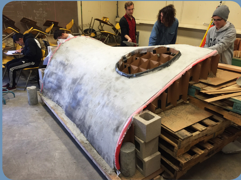
CURED CONCRETE SHELL
