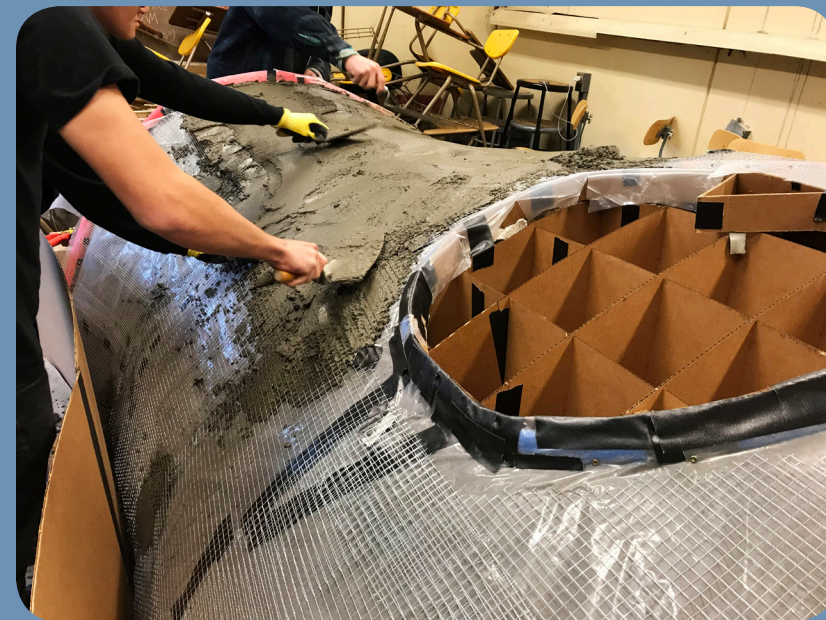
CONCRETE IS APPLIED WITH WIRE MESH AS REINFORCEMENT
