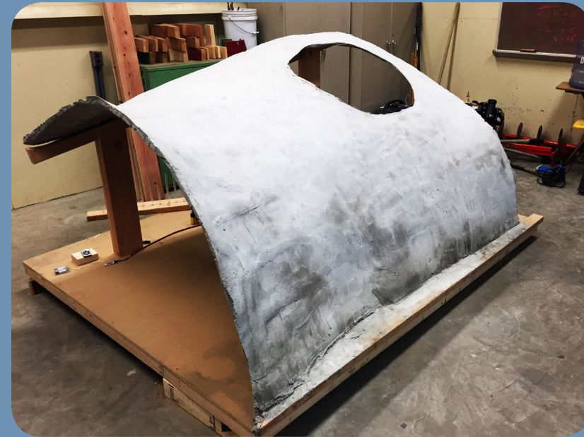
FORMWORK REMOVED AND SUPPORT BEAMS ARE PLACED
