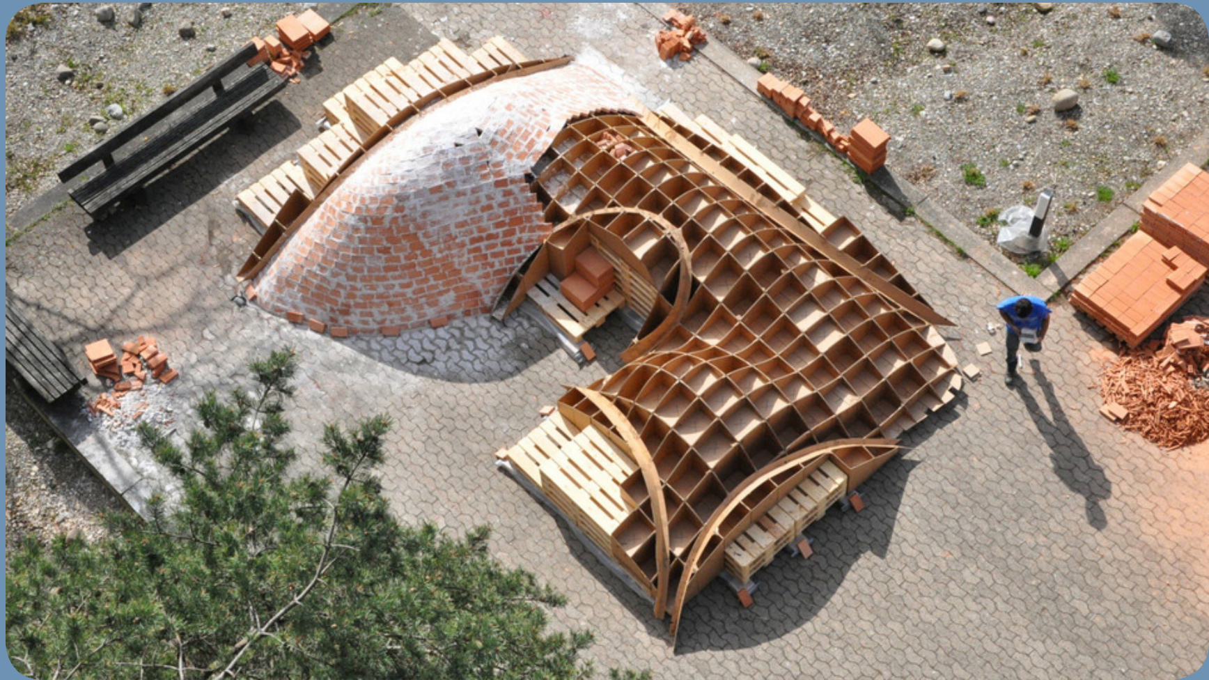
FREE-FORM CATALAN VAULT ZURICH, SWITZERLAND
