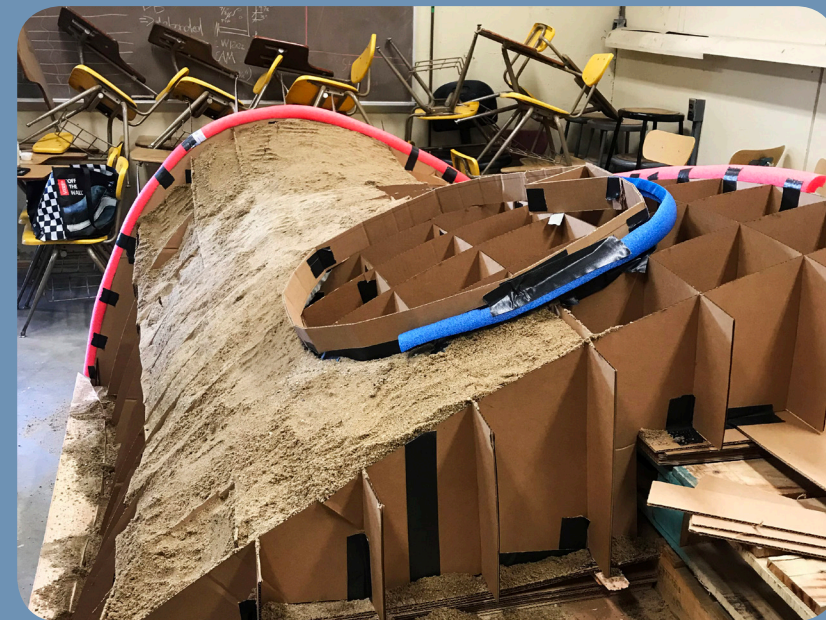
ATTACHED EDGES TO RETAIN SAND
