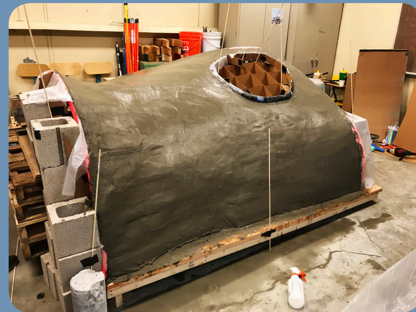
CONCRETE IS SMOOTHED AND FINISHED FOR CURING
