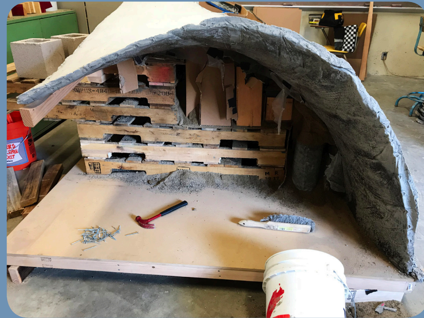
FORMWORK REMOVAL
