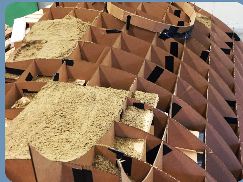
FILLING WAFFLE VOIDS WITH SAND
