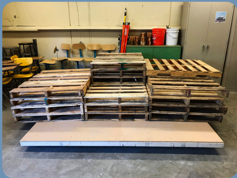
PALLET SUBSTITUTION FOR SCAFFOLDING
