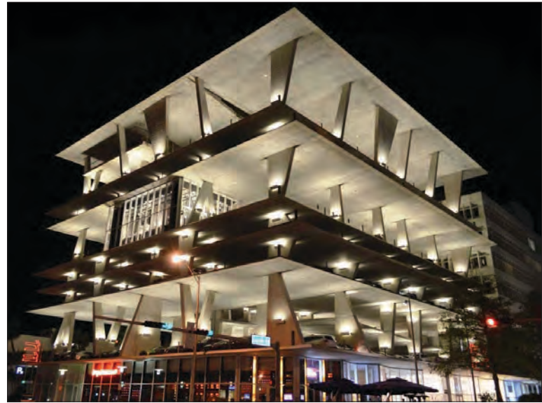
Figure 15: This parking structure in Miami, designed by Herzog & de Meuron, is also used as an event space in the evenings and weekends. (source: www.dssconsultants.com )
