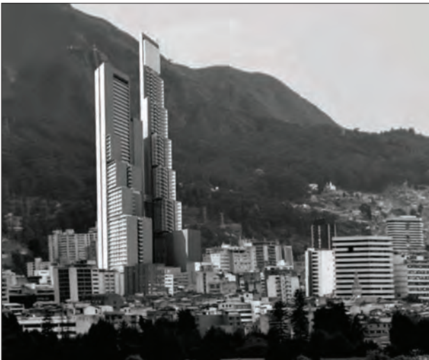
Figure 17: Bacata Complex in Bogotá, under construction through crowd sourcing. (source: www.bdbacata.com )
