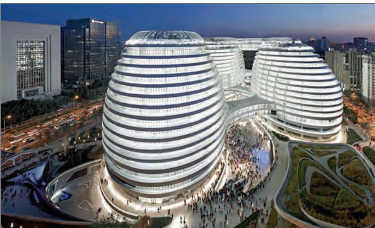
Figure 18: Zaha Hadid's Galaxy complex in Beijing. Innovative design relying on hundreds of large and small investors. (source: http://ideasdesign.today )
