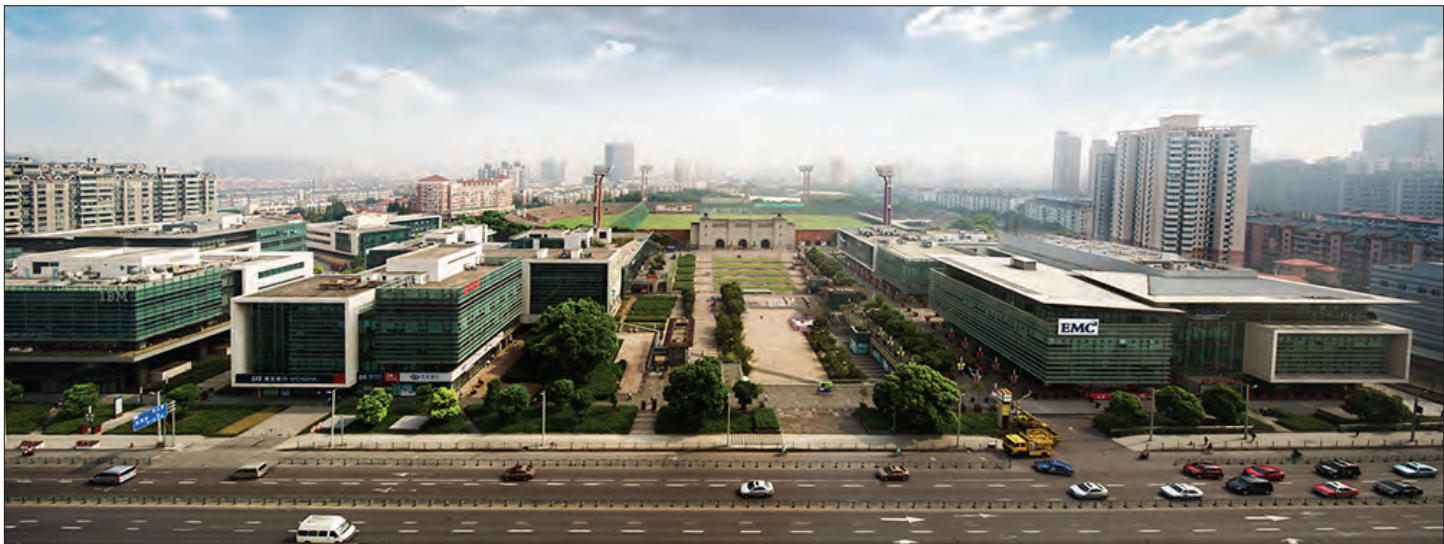
Figure 12: In Shanghai, the Knowledge and Innovations Community is a high-tech R&D and live-work development next to a university district serving several institutions. (source: www.casestudies.uli.org )
