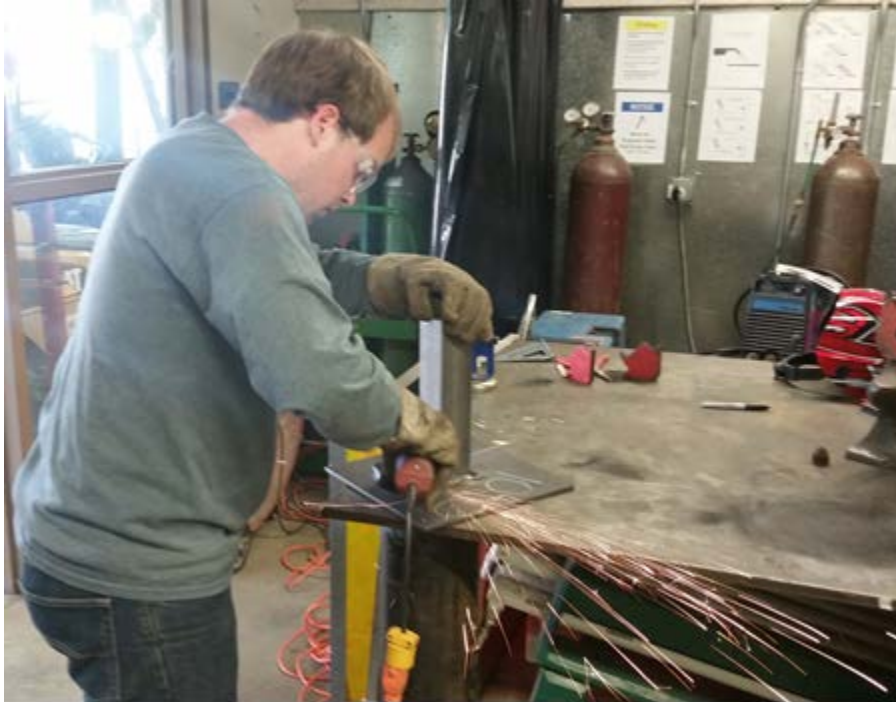
Figure 6.1.5. Finish Grinding of Welds.
