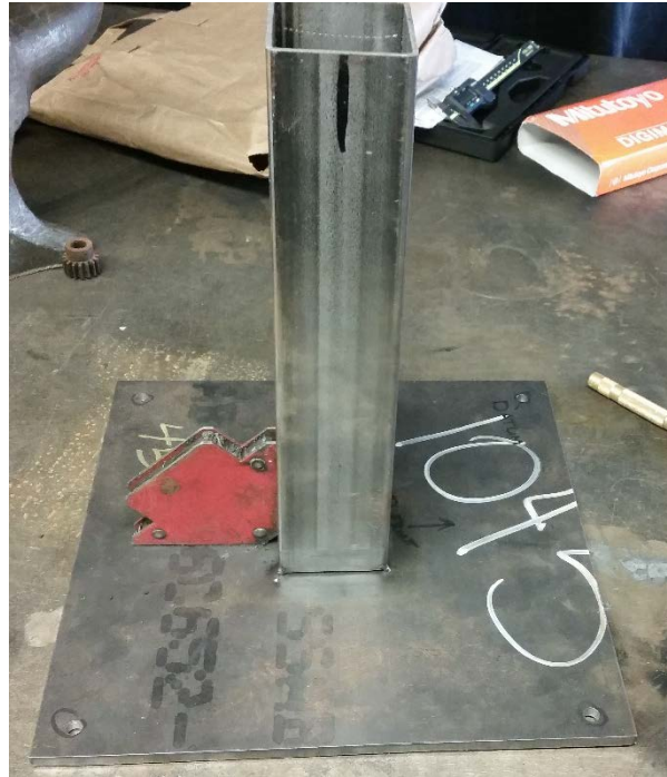
Figure 6.1.2. Vertical Lower Tube ready for welding.
