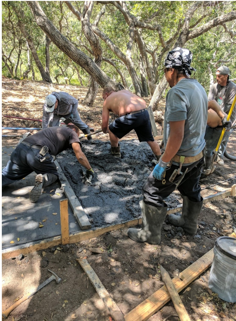
Figure 8: Jordan Pumping Pouring Sidewalk
