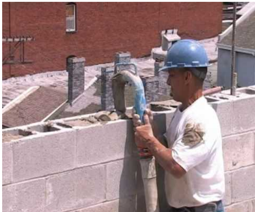
Figure 2: Grout Pumped into Masonry Wall
