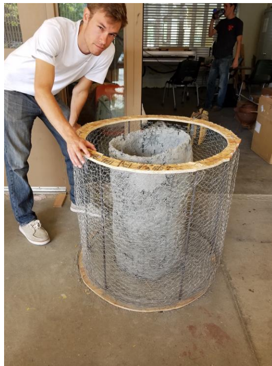
Figure 32. Kyle poses with the improved mesh and rebar backbone of the outer housing walls.
