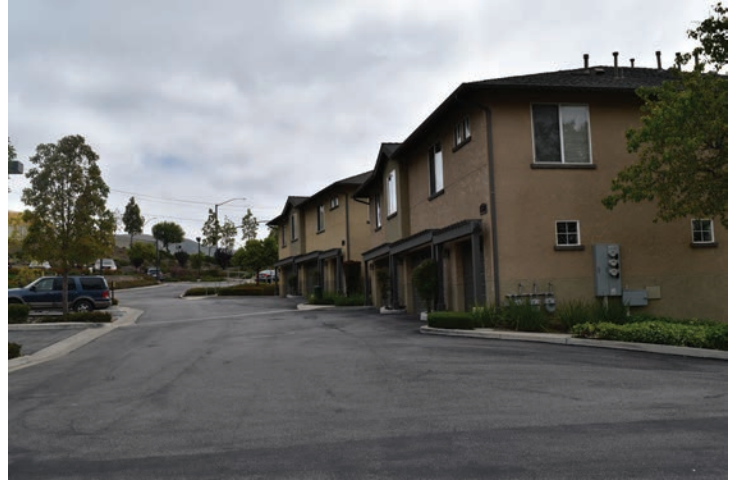
Existing conditions at Bella Montana
