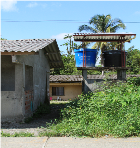
Figure 6.2 – Containers to collect rainwater in Bajo Calima, Buenaventura (photo credit: Bayeté Ross Smith)
