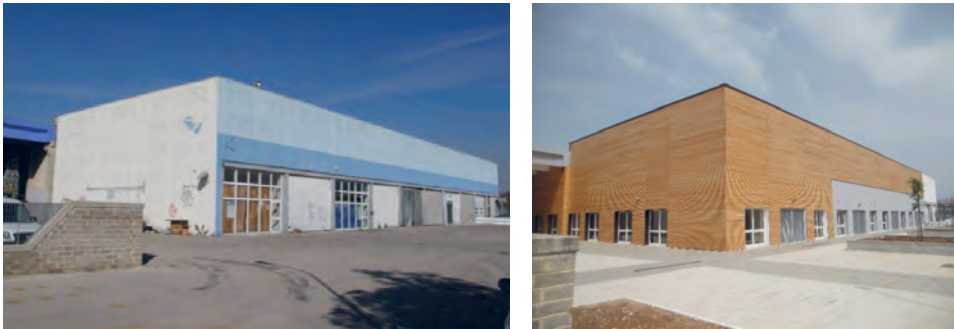
Fig. 5. The “Ex-Claudia” plant, before and after the works
