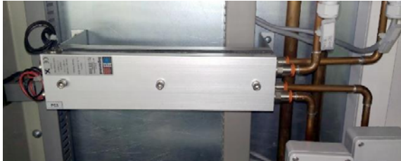
Fig. 6. Thermoelectric assembly type L.L.-210-24-00-00.
