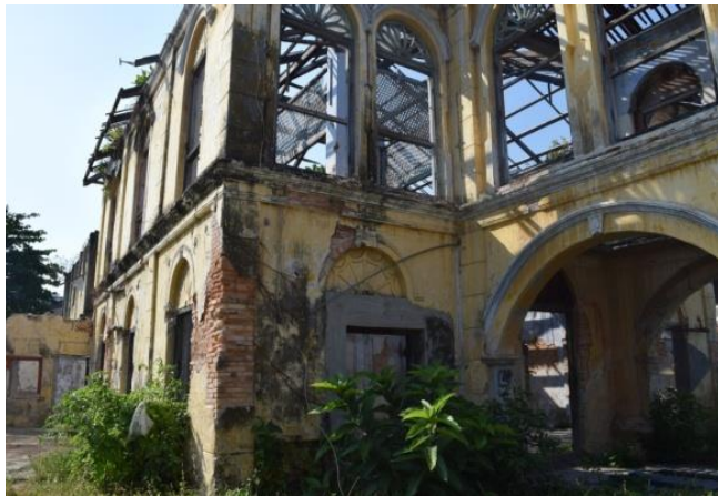
Figure 8. Doubled-storey Mansion at Jalan Dato Koyah
