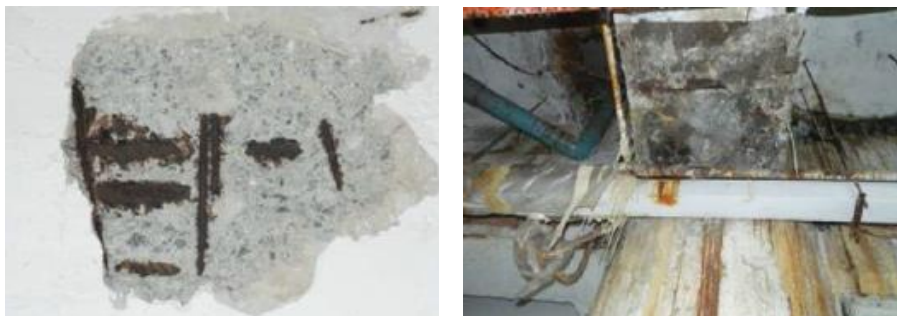
Figure 9. The condition of structure inside the M&E room
