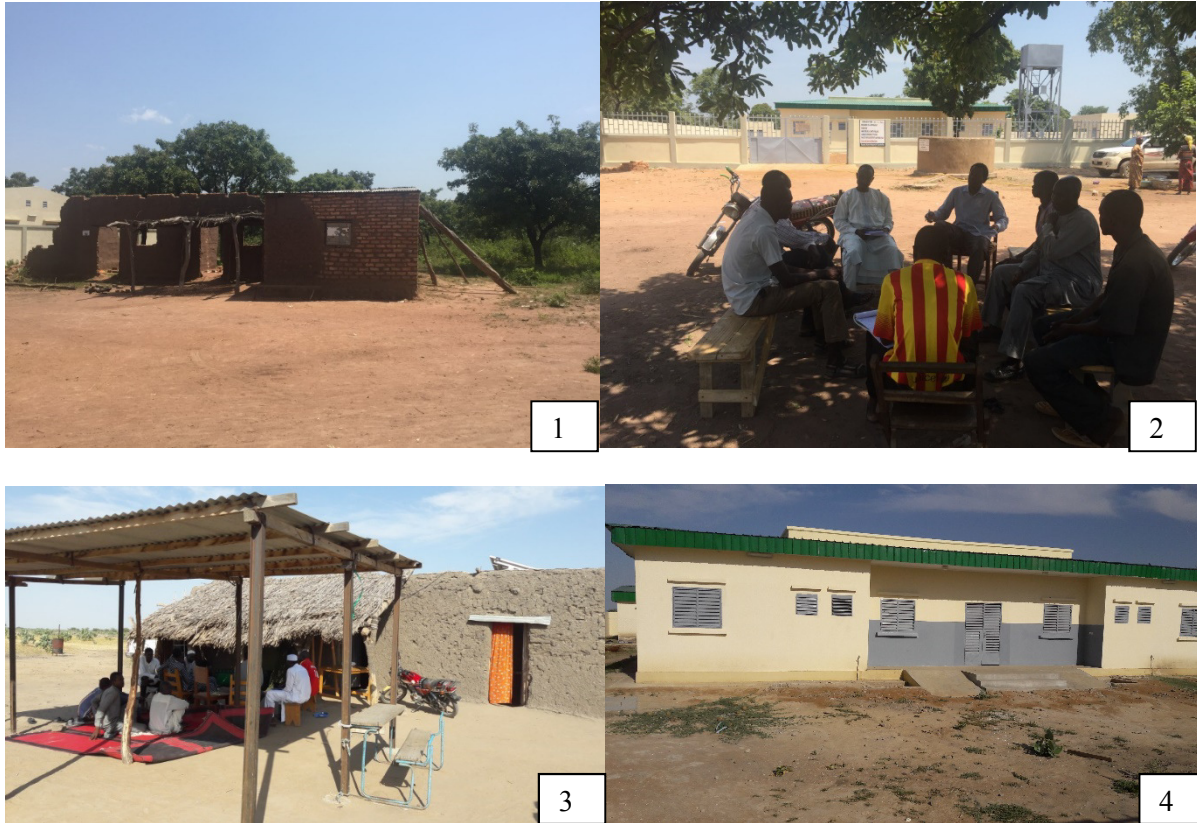
Health infrastructures: old health centers (left) and newly constructed health centers by PADS (right) in Danamadji (Djeke-djeke 1 & 2) and Yao (Abregna-breka 3&4) health districts
