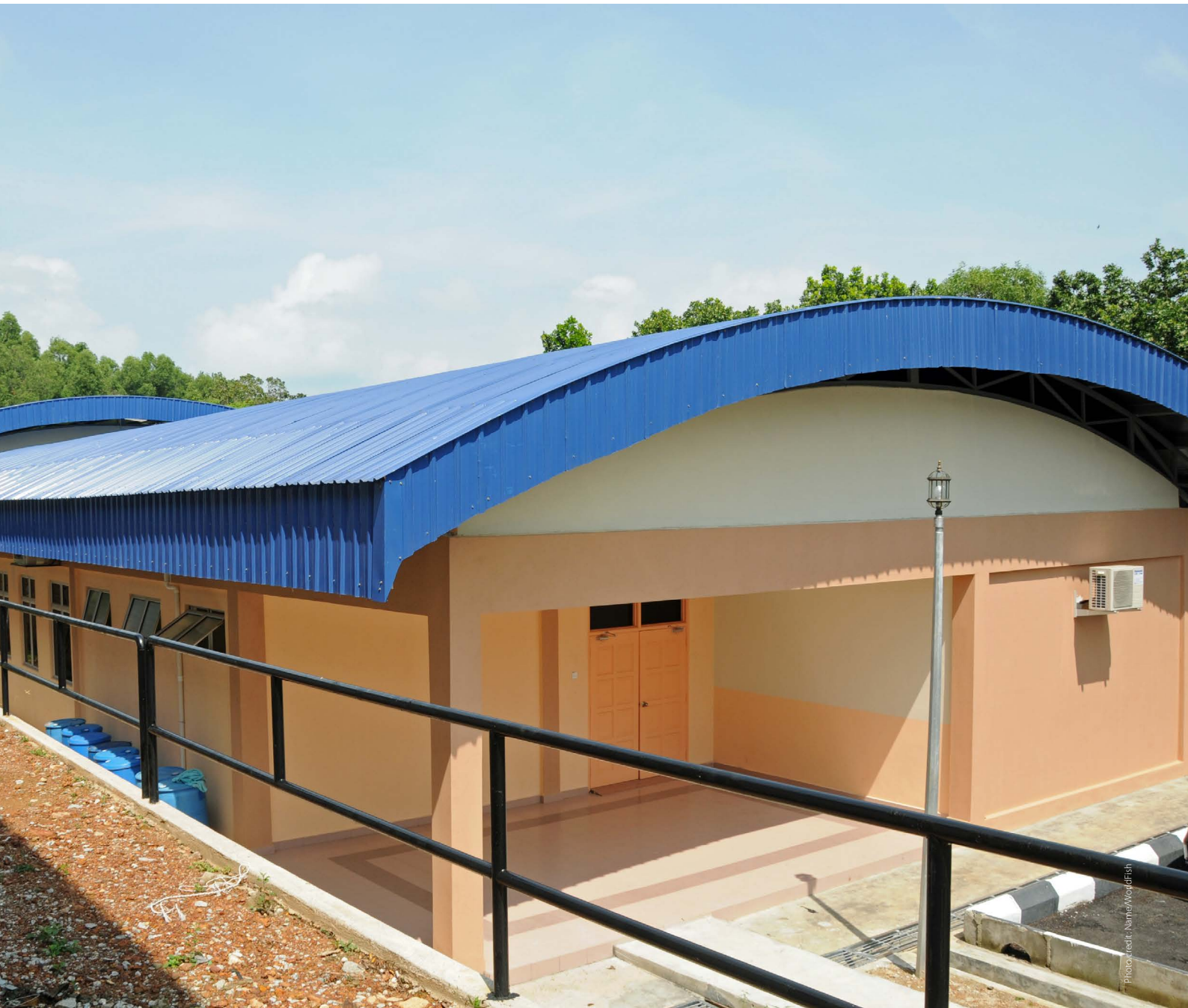
Good example of a closed up hatchery to reduce the risk of introducing pathogens.
