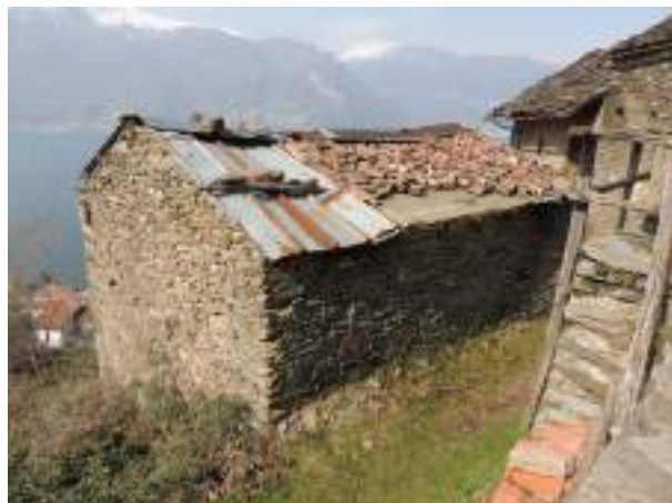
Fig. 18 - Same technique to form a railing to contain stones, but with a new material. (photo: Andrea L'Erario)
