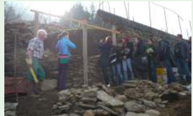
Fig. 27 - Look at the structure to help follow the alignment and the arrangement of stones at the foundation of the wall. (photo Alessia Silveti)
