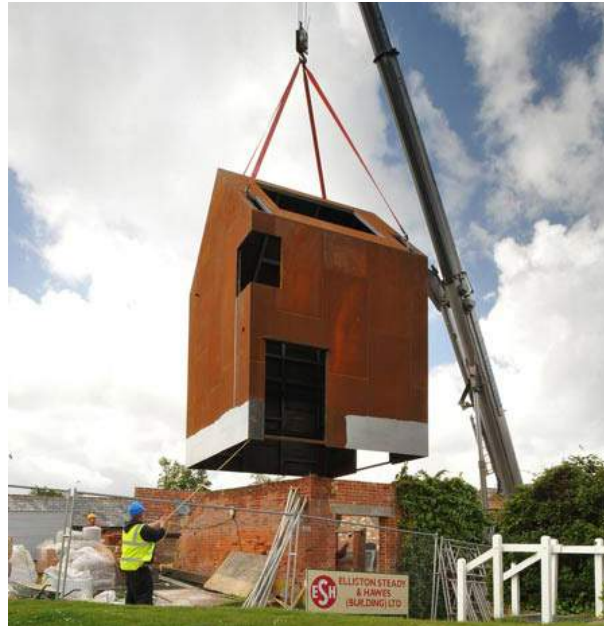
Fig. 5, 6 and 7 - Dovecote Studio by Haworth Thompkins, Suffolk, England, 2009 (source: www.archdaily.com )
