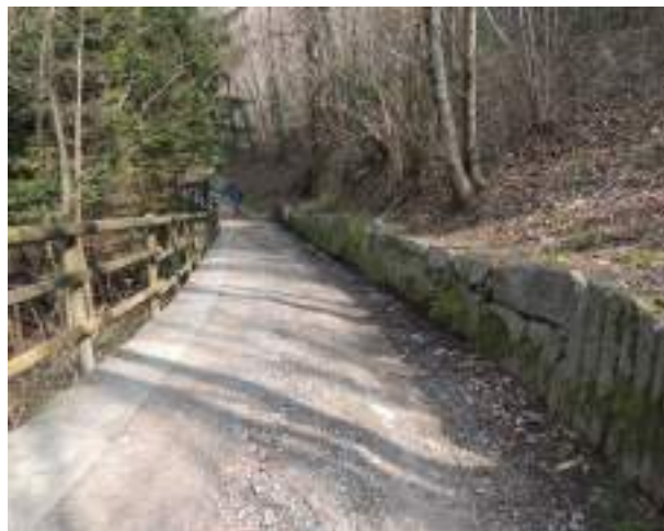
Fig. 6 - The Viandante pathway in the south part from Mondonico to Dervio does not conserve historical characteristics: dimensions have been changed for being vehicle accessible and historical elements now include concrete reinforcements. The new wood railing is too smooth and its forms belongs to wood industry not handcrafted production. (photo: Andrea L'Erario)
