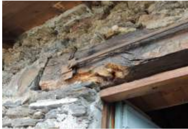
Fig. 16 - Reinforcement of a beam with a new material. (photo: Andrea L'Erario)
