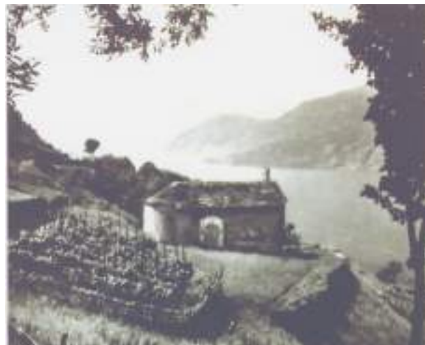
Fig. 7 - Saint George Church, north-eastern elevation. On this side, another small volume is visible, probably the a chapel. (source: Alfonso Piva)
