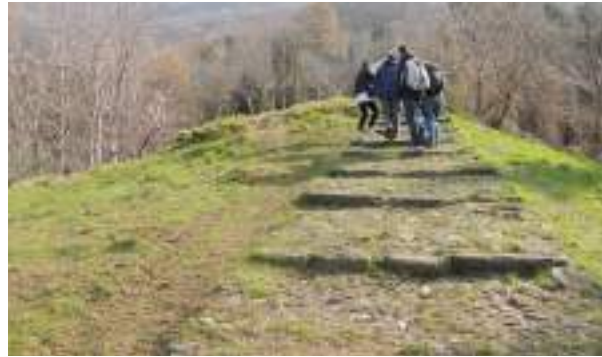
Fig. 3 – The historical paving, made by stones and pebbles, still characterizes the Heritage path . It is important to maintain this kind of pavement to keep the path identity (photo: Andrea L'Erario, 2014)
