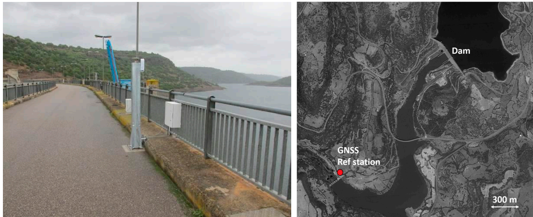
Figure 3. One of the GNSS antenna monitoring the dam and the position of the reference station.
