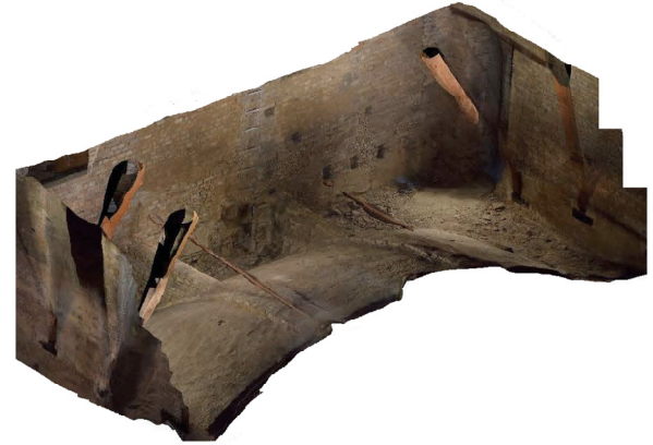
Figure6. The 3Dorthoimage of the intrados obtained on the laser-scans GCPs of the vault (upper); the 3D orthoimage of the extrados obtained by the photogrammetric image block (bottom). (© GICARUS lab, PhD Riccardo Valente, and students courtesy).
