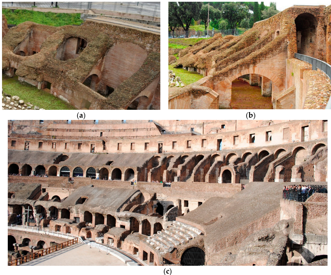
Figure 7. Examples of the structure built as a support of the podium with a double purpose, upholding the structure of the seats and corridor for the public to reach their seats: (a,b) Circus Maximus in Rome; (c) Flavian Amphitheatre (Colosseum) in Rome.
