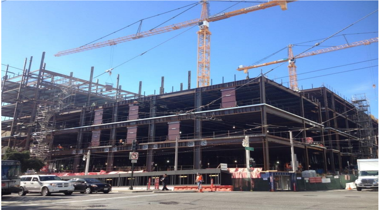
Figure 45. Van Ness and Geary Hospital construction site visited in December 2015.
