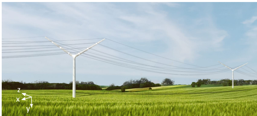
Figure 1: Composite power pylon with directly attached overhead transmission line bundles in the global coordinate system [15].
