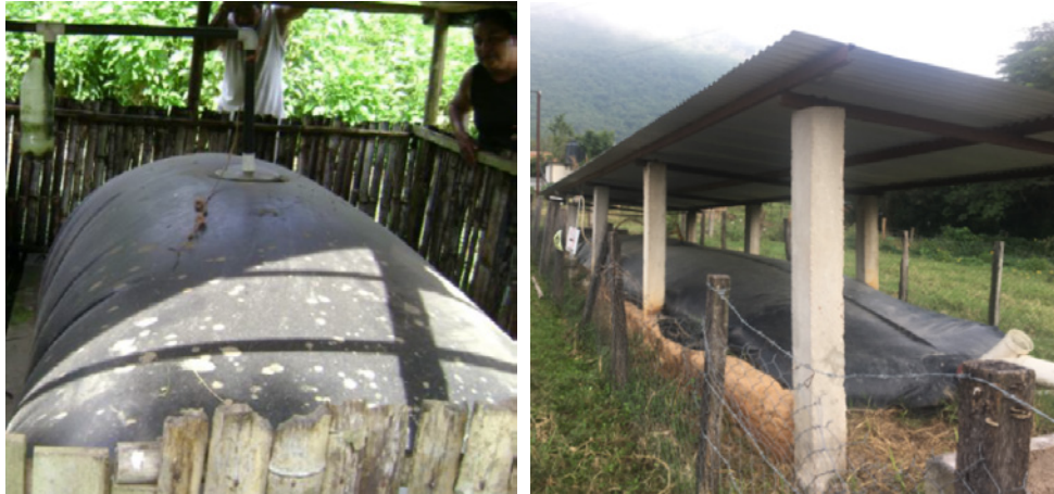
Figure 10. Low-cost and medium-cost family biodigesters
